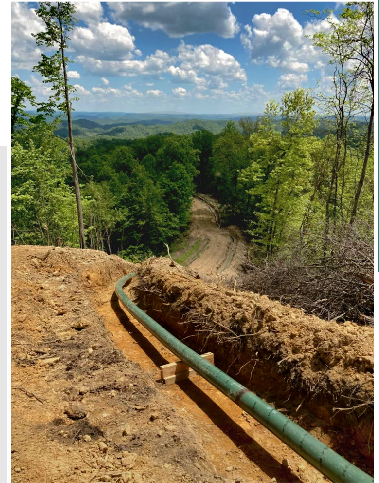
Company Image: Installation of new transportation pipeline
