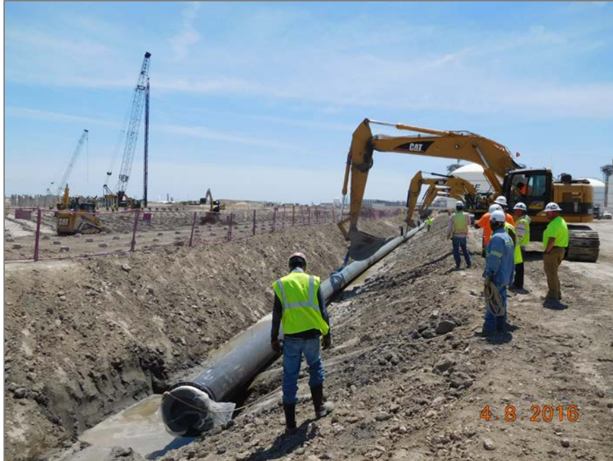
Train 5 – Installation of West Ring of ISBL Firewater Pipe
