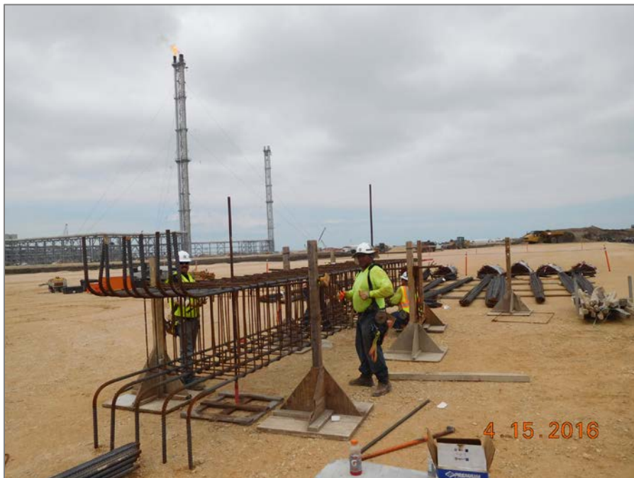
Train 5 - Prefabricating Rebar for Compressor Deck Columns
