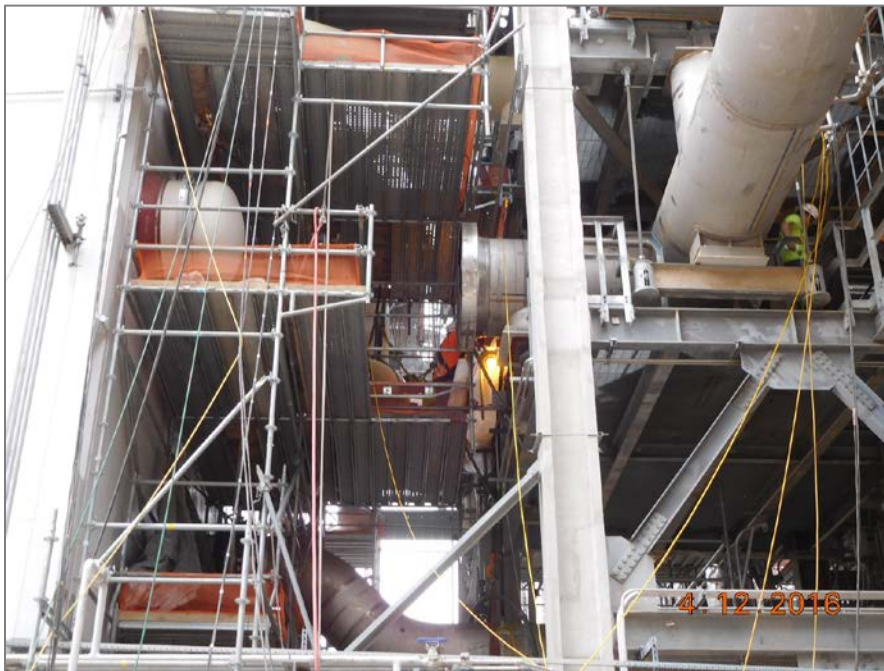
Train 2 - Installation of Aboveground Pipe Connections to Ethylene Cold Box
