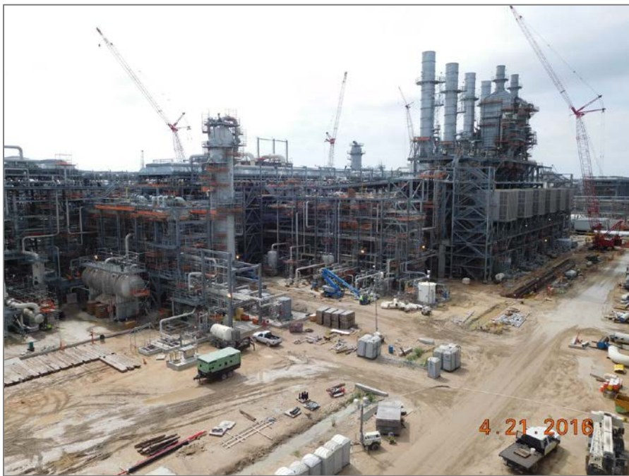
Train 3 - Overview from North West
