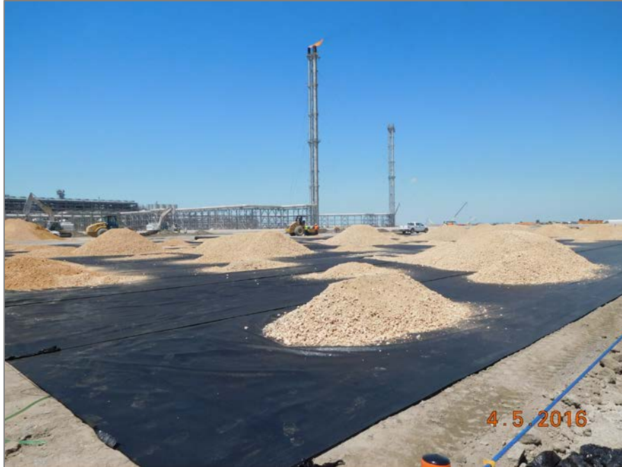
OSBL - Final Grading of Common Areas West of Stage 3 Flare Rack
